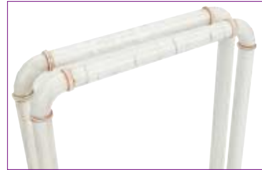
Dirty Pipe Joints
