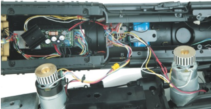
Figure 14: Boiler Wire Harness
